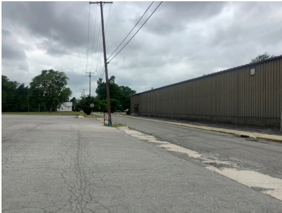
Photo Location 3. View of industrial habitat. Photograph taken facing east.
